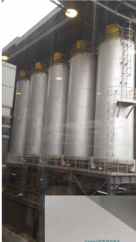
Tank for incineration residue
