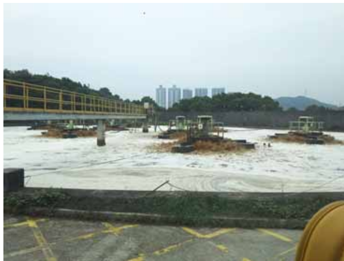
Leachate treatment systems
