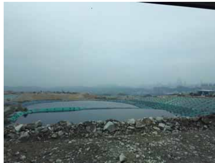
Leachate reservoir on landfill site
